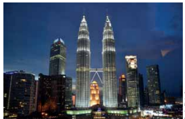
Malaysian oil and gas giant Petronas is even considering solar power through a new unit.
