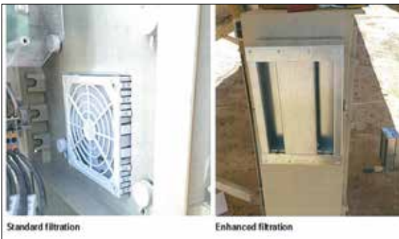
Figure 7. Standard versus enhanced array box filtration
