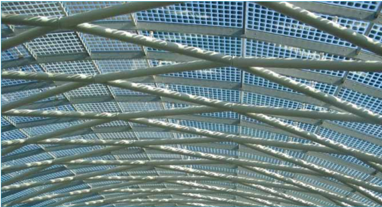
Figure 2. Romag's BIPV installation in the London Borough of Hackney, UK, covers the glazed roof of the local Council's 'Customer First Centre'.
