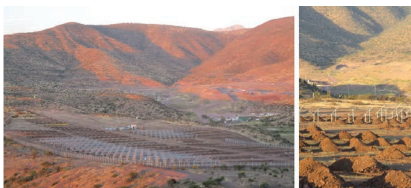
Figure 8. The bifacial PV system currently being set up by MegaEngineering and Imelsa. With a total power of 2.5MWp and 3.25MWpe [15], the 'BiSoN farm' will become the world's largest bifacial PV system.
