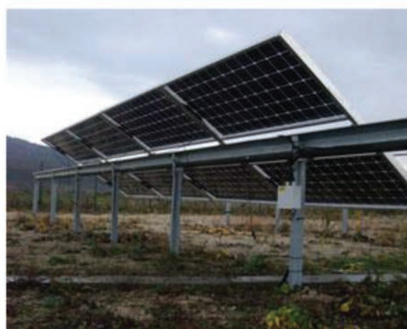
Figure 6. Commercial open-field installation in Saxony, Germany: 8 months with a 20% (0.2) reflectance ground albedo and 12 months with a 50% (0.5) reflectance ground albedo. Results: 17% bifaciality gain over the best module in the field and more than 60% gain in snowy conditions. (The bifacial system kept collecting solar energy through the back side even when the front side was covered with snow, in contrast to all the other systems, which stopped yielding power in these conditions.) The respective cell equivalent efficiency values are 21.7% and 29.6% [13].
