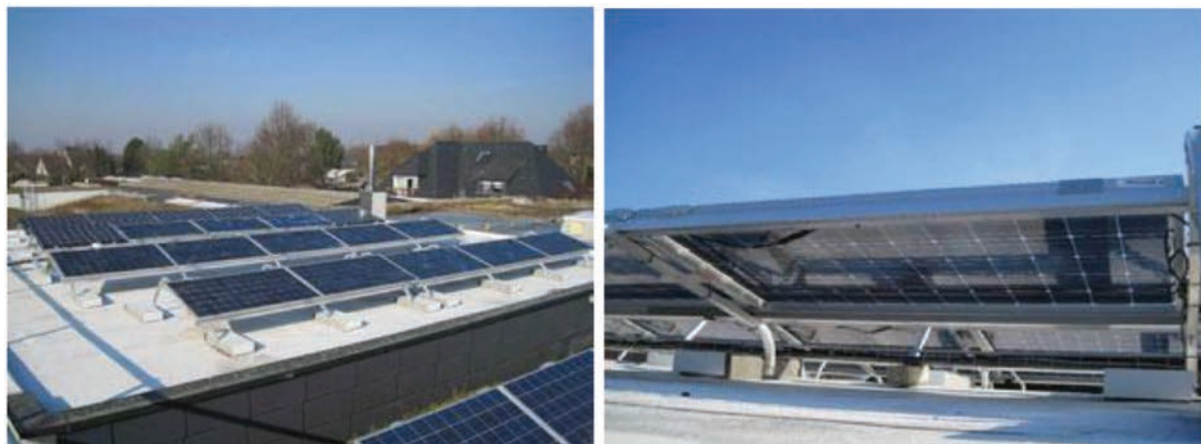
Figure 10. A commercial installation in Geilenkirchen, Germany, monitored by Fraunhofer/ISE (20cm height above the rooftop, 78% reflectance white roof membrane, nine-month period). Results: bifaciality gain = 21.4%; effective cell efficiency = 22.5% [13].v
