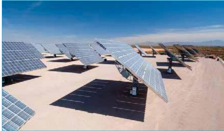
Tracking the desert sun, a 2MW array of Amonix CPV systems generates clean electricity at the science and technology park at the University of Arizona (Tucson, AZ, USA).
