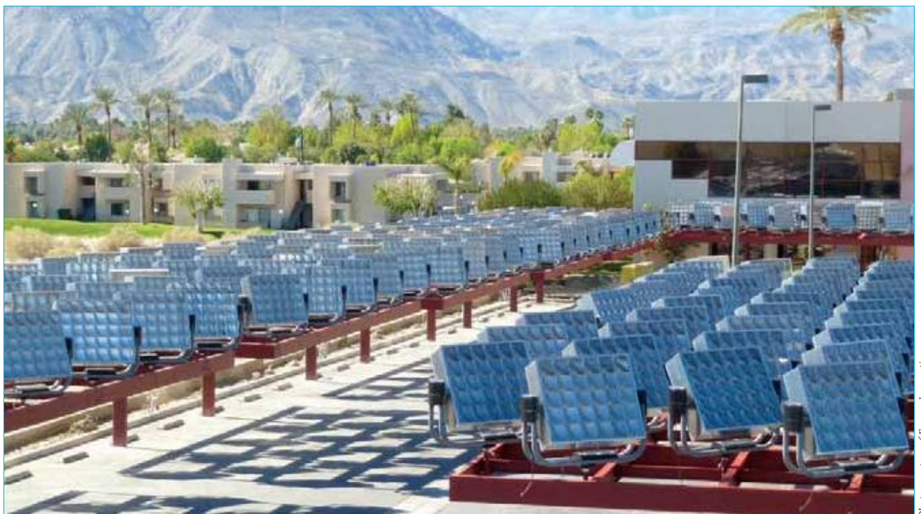
At a 600kW project in Palm Springs, CA, USA, Energy Innovations is deploying both carport and field-mounted CPV systems.
