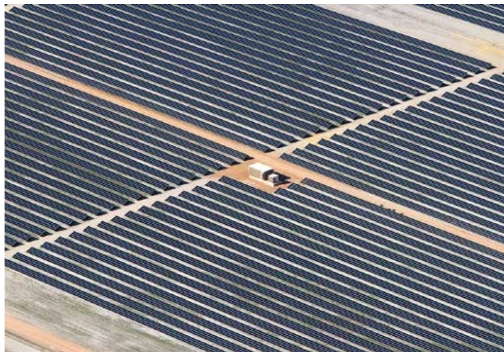
Credit: First Solar
