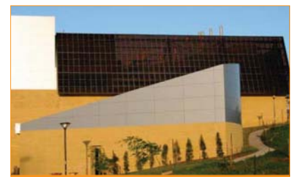
Figure 6. Dyesol manufactured the solar wall panels to supply and install in the CSIRO Energy Centre in Newcastle, Australia.
