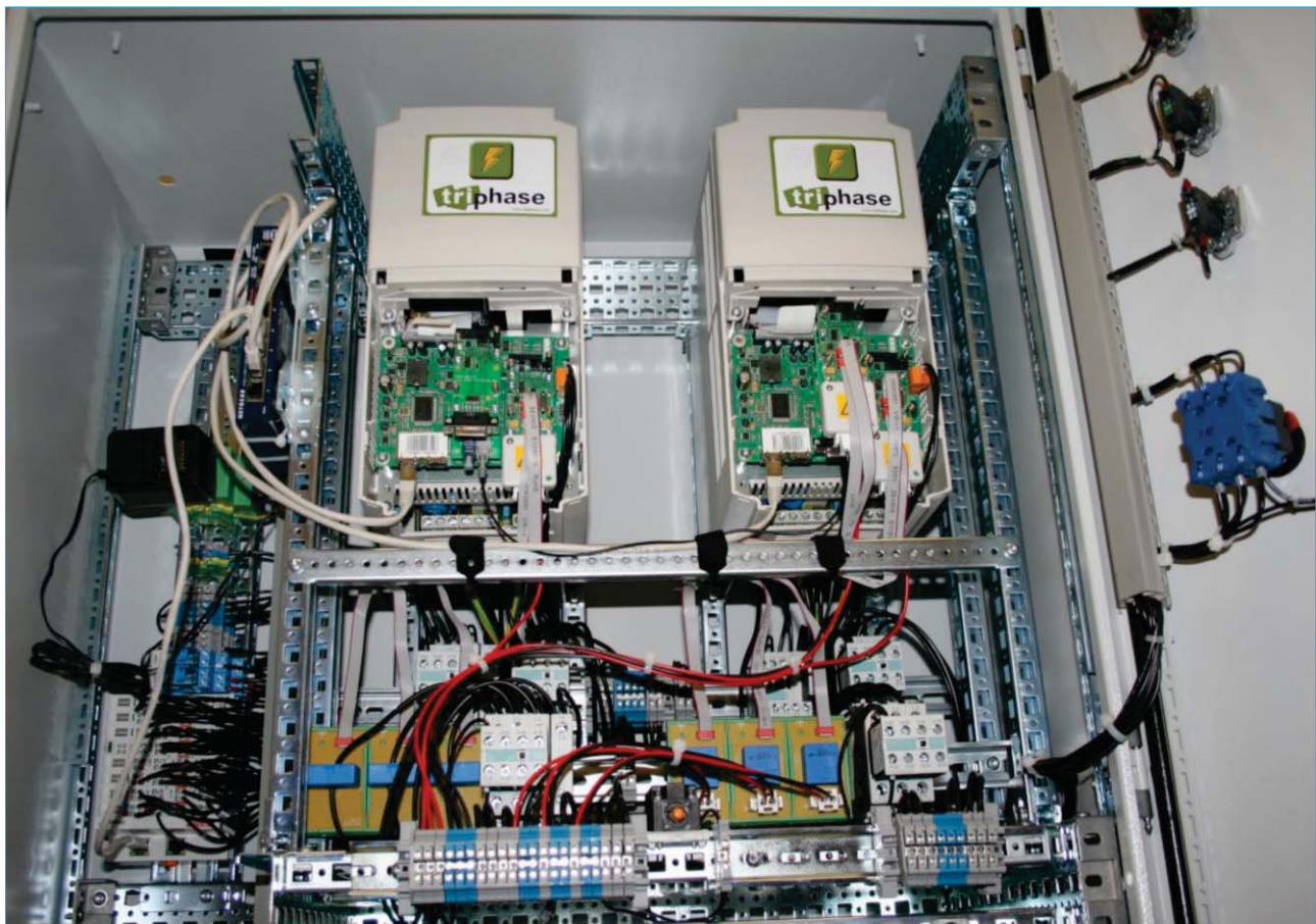
Figure 3. Internal view of a power electronic system coupling a distributed energy resource and storage units to the grid.
