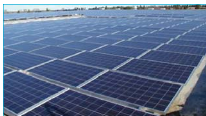
California commercial rooftop installation.
