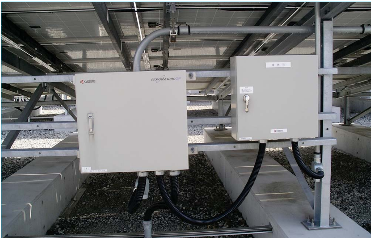
Figure 1. Inverters installed in the shadow of a PV array.
