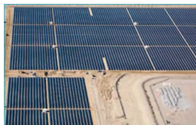
First Solar selected for Masdar City project.
