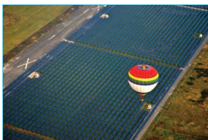
juwi's installation at Waldpolenz solar park.
