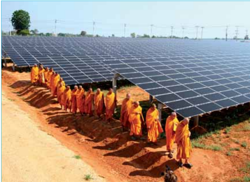
A 7.5MW solar plant worth €22.8million has been built in the north-west province of Nakhon Ratchasima, Thailand.
