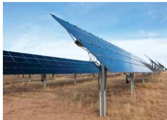
Credit: First Solar
