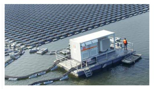
Sungrow also set up its own transmission lines from the floating matrix to the booster station and then to the gridconnection point. Power from the project is also being sold to utility State Grid Corporation of China (SGCC).
