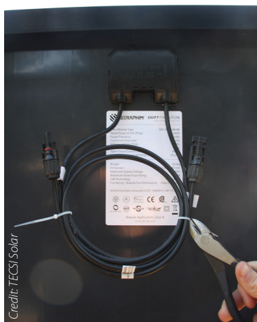
Figure 12. Removing standard factory installed wire ties
