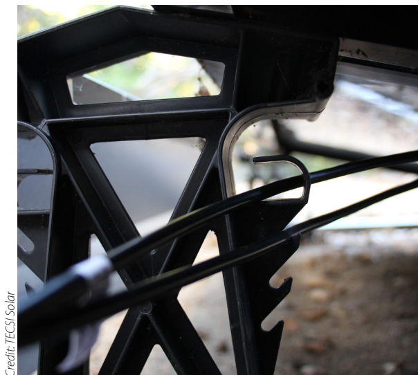
Figure 8. Esdec racking integrated wire management
