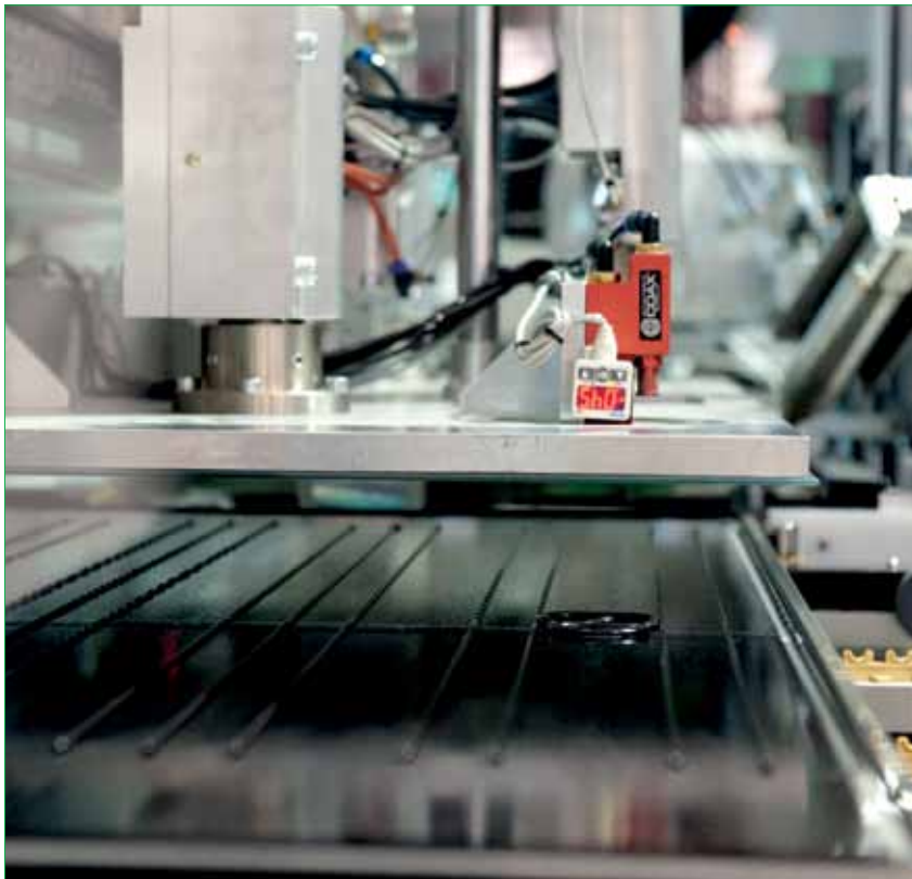
Figure 10. Desiccated PIB dispense station on a manufacturing line.
