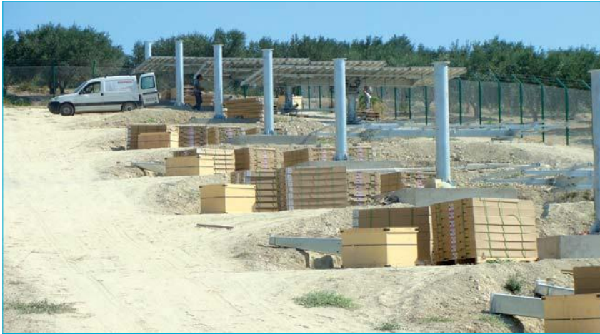
The SolFocus-equipped CPV power plant project under construction in Crete.
