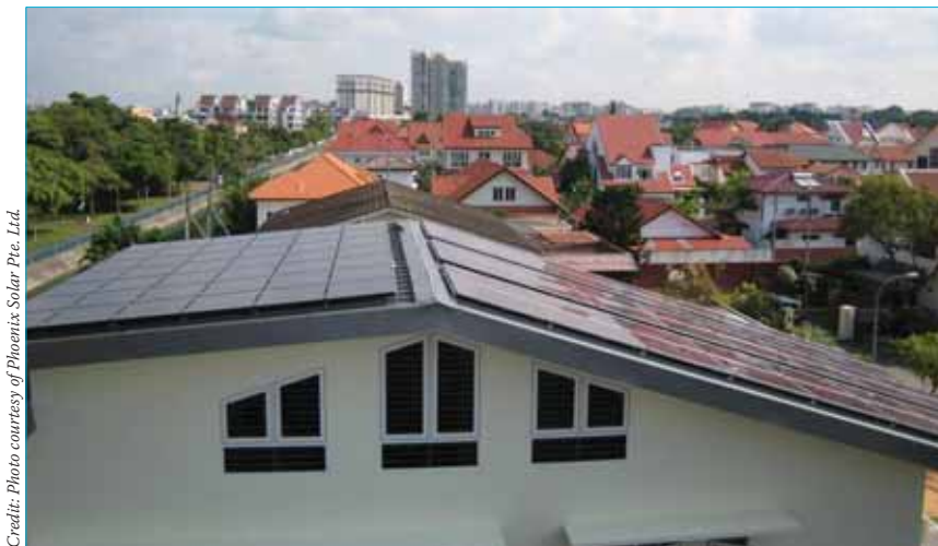
Figure 6. The first zero-energy house in Singapore: the east-facing roof is tilted at 18.3° (right side of the roof), while the west-facing roof is tilted at 6.1° (left side of the roof).
