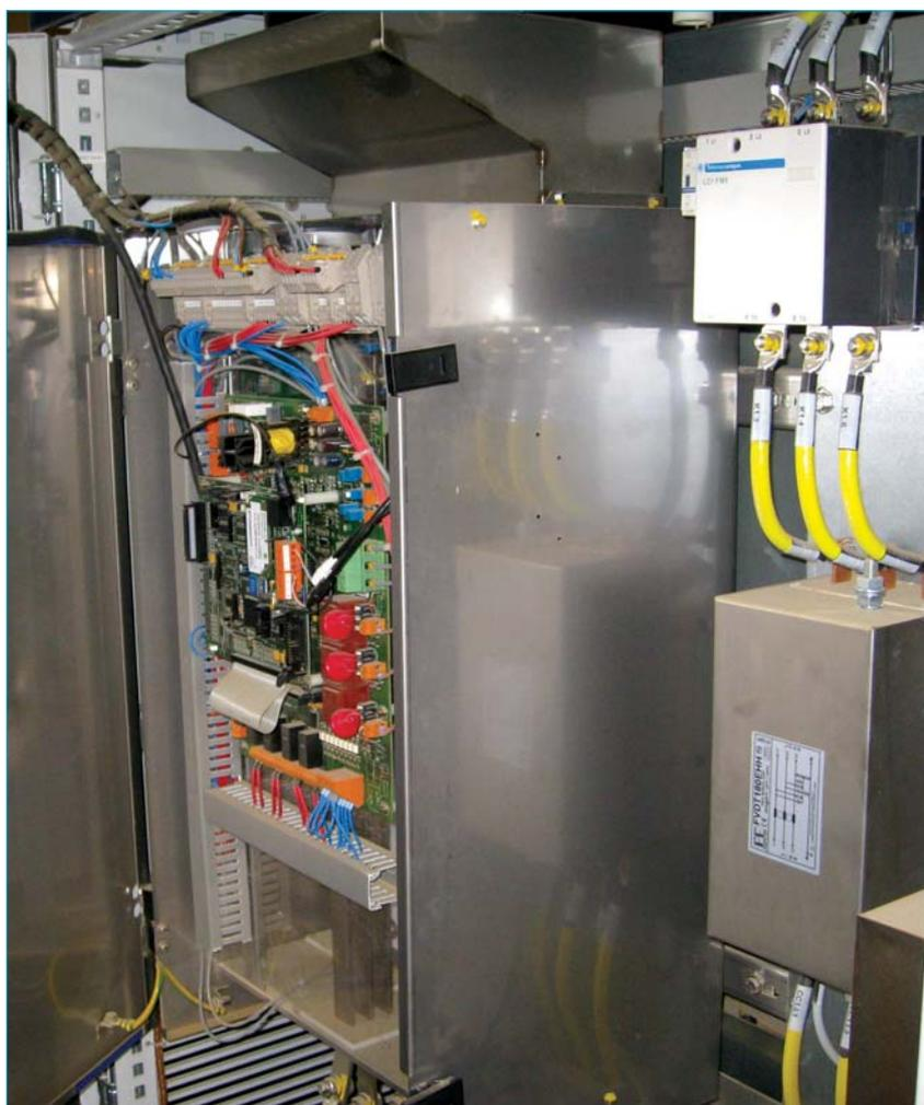
Figure 1. A PV grid-connected inverter installed in a Spanish PV plant.
