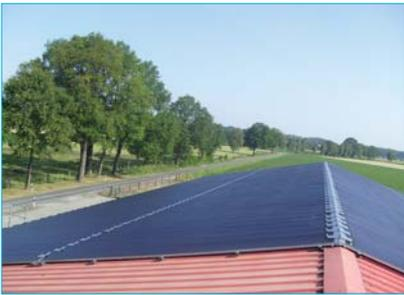
**Centrosolar offers trapezoidal roofing solution for flexible thin-film mounting**
