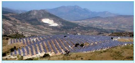
Location: Jaén, Spain Nominal power: 2.1MWp Trackers: 906 Ground area: Approx. 150,000m<sup>2</sup> Solar modules: Approx. 10,600 units Electricity production: Approx. 4,000,000kWh per annum Completion date: July 2008 Involvement: Concept, Detailed Engineering, Project Finance, Licensing, Negotiations with Public Administrations, Supply Chain, EPC, Optimization, 0&M.
