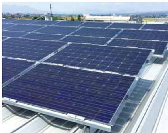
level AC/DC ratio of 0.95+ reduces LCOE and boosts lifetime yield. The GxB380 SM offers increased flexibility, as modules with optimisers can be easily installed with complex rooftops or shading from trees, chimneys and other obstructions.
